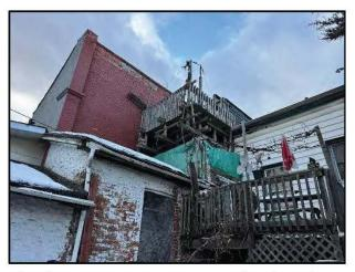
conventional wood framing atop the exposed earth. The superstructure appeared to have been supported on a cast in place concrete foundation.
