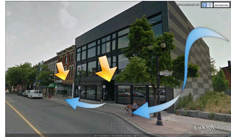
Image 10 - Recessed Entrances to Existing Buildings (Photo Courtesy of Google earth™)
