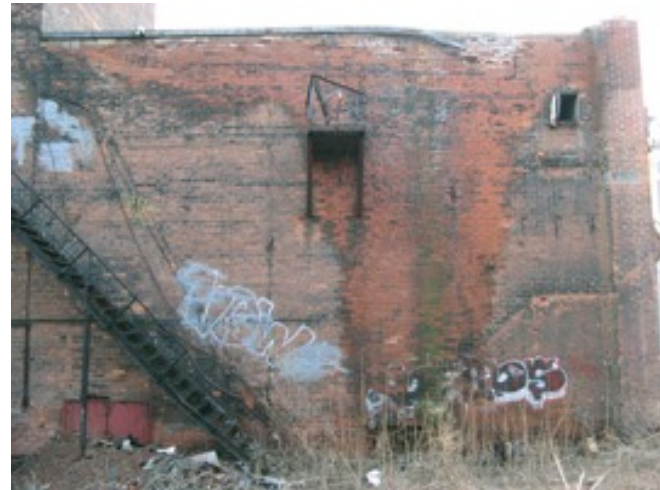
North Side of concourse, not roof flashing ripped off at west, right, end of roof
