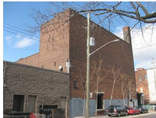
General view of east wall. Note location of deteriorated chimney
