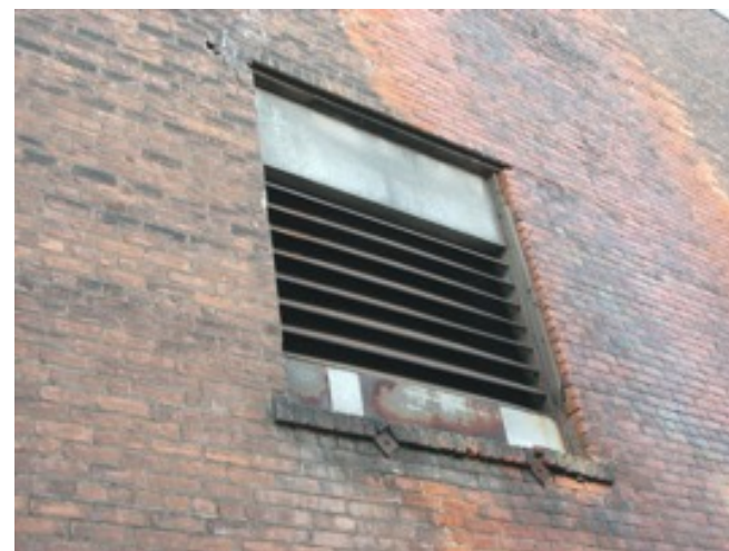
Detail existing Grille on north wall. This can be used to ventilate the interior
