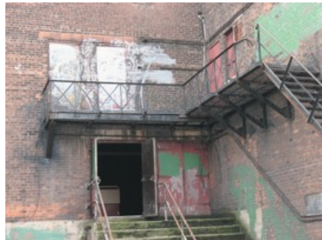
Doors to auditorium and projection room. These should be sealed up, use concrete block or brick which may be removed in future.
