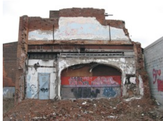
Detail at cut of concourse, a new exterior wall is required to seal this location against weather and vandals.
