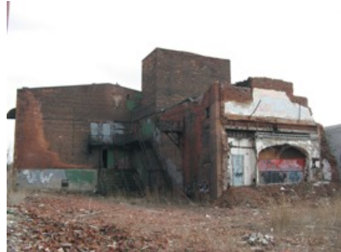
West elevation of remaining building showing concourse cut off with auditorium house beyond
