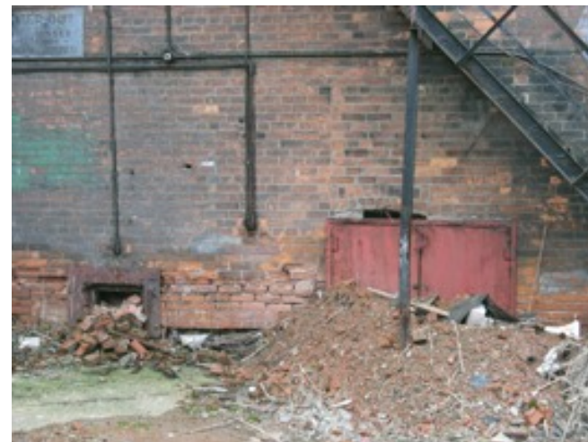
Detail at north wall of concourse, note open hatch to crawl space admitting water and vandals, partially blocked by loose masonry at present.
