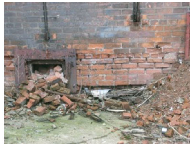
Detail at north wall of concourse. The brick masonry is severely deteriorated in this area and one full wythe of brick is missing. Joints should be pointed and missing brick replaced.
