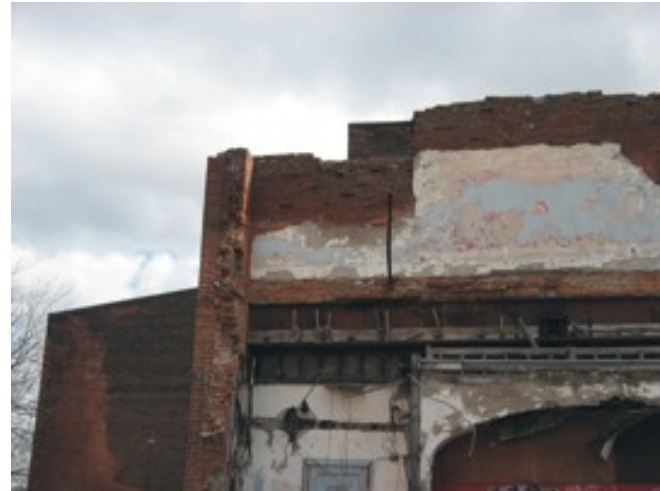
Detail at concourse, no roof flashing or roof seal at concourse
