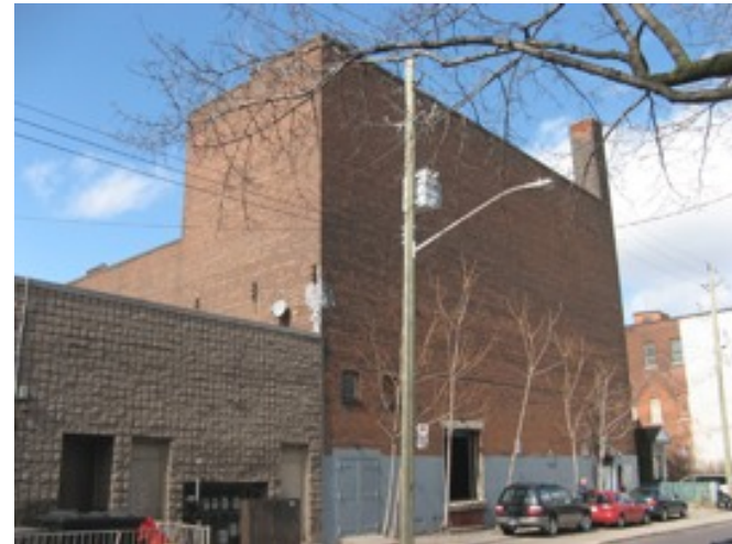
East Elevation, rear, of the building showing stage house
