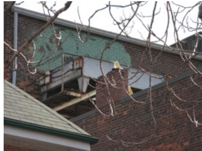
Detail of brick pier at north side of auditorium. This supports roof top equipment and should be repointed and missing bricks replaced.
