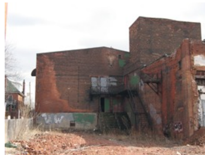
West end of auditorium house, staining indicates where water flows off flooded roof. This also flows to the interior under the roof flashings
