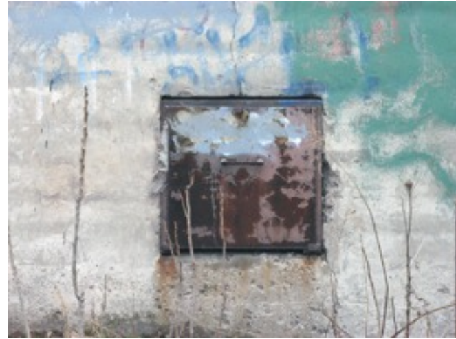
Example of access hatch. There are several around the building. An attempt to pry this open is apparent. These should be further secured and sealed against the weather.
